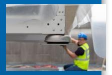
▲ With a sound insulation mat in between, the steel frames are screwed to the concrete bases, and the JAEGGI ADC units in turn, placed on sound insulation legs, are mounted on the steel frames
