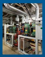
▲ When the waste heat of the CHP is not required for the raw water and heating during summer, it is used as energy source for the absorption chiller
