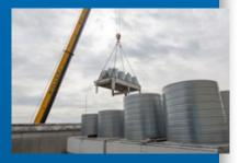
▲ Before issuing the invitation to tender, it was already evident that the cooling capacity on the "balcony", packed with twenty-year-old Güntner flat bed coolers (4 x 130 kW/4 x 444 MBTU/h), was not sufficient.
