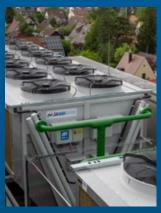
▲ Both JAEGGI ADC dry cooling units, connected in parallel, are controlled via a Güntner Motor Management system as well as a Hydro Management system and a superordinate Güntner Master Panel that is connected to the building management system.
